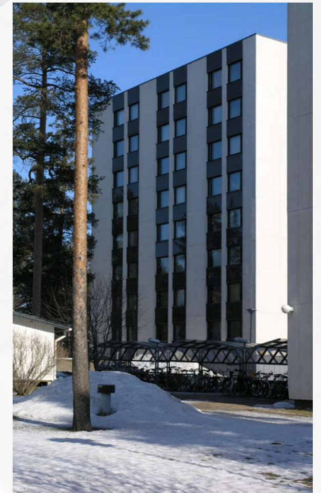
The renovation of Pohjankaleva building aims at reaching the Finnish Passive House level, where the heating energy demand after renovation is max. 30 kWh/m 2 /a. The location of the Oulu pilot building is 65° 02' N
